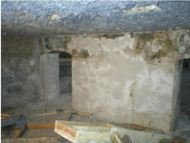
**Figure 7. Hot wall installation with forms stripped**
